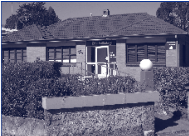
The new Toowoomba Laboratory Scott St, Toowoomba
